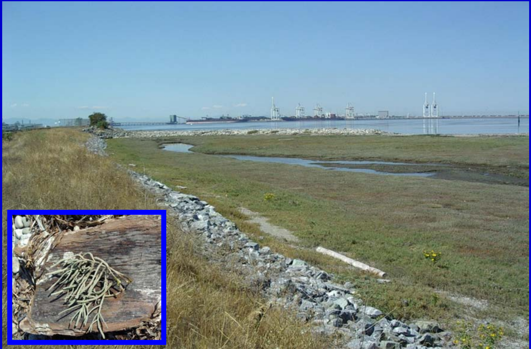
CONSTRUCTED SALICORNIA MARSH – NEAR BOUNDARY BAY, BC
